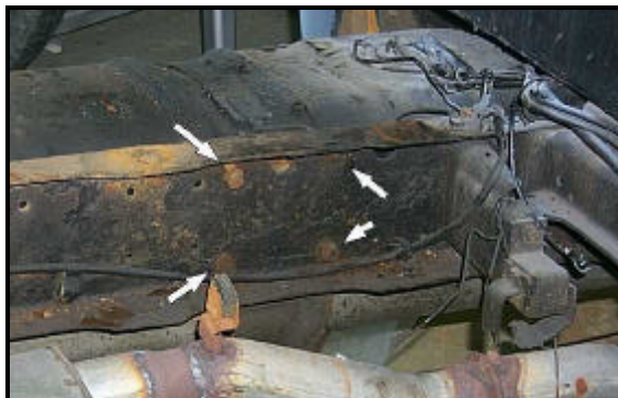
Figure 2: Bolts attaching the rear tank brackets to the frame rail.
